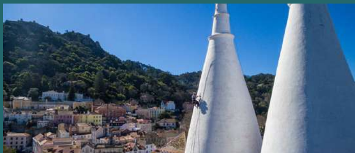
Maintenance action with the use of lime. Photo by Parques de Sintra, Monte da Lua.
